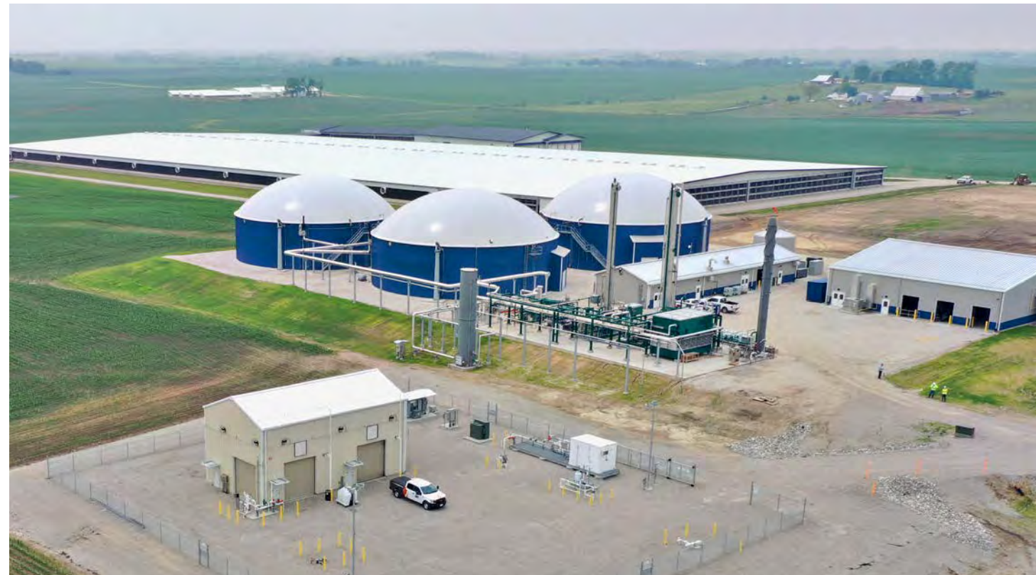
Marshall Ridge Dairy renewable natural gas partnership — Pictured: manure anaerobic digesters and Black Hills Energy's renewable natural gas interconnection
